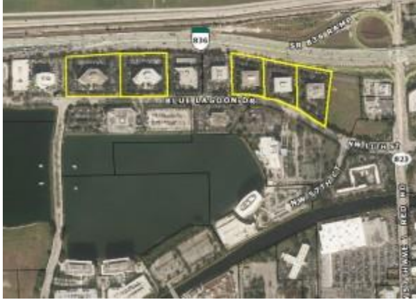
Aerial view of the five buildings included in sale
